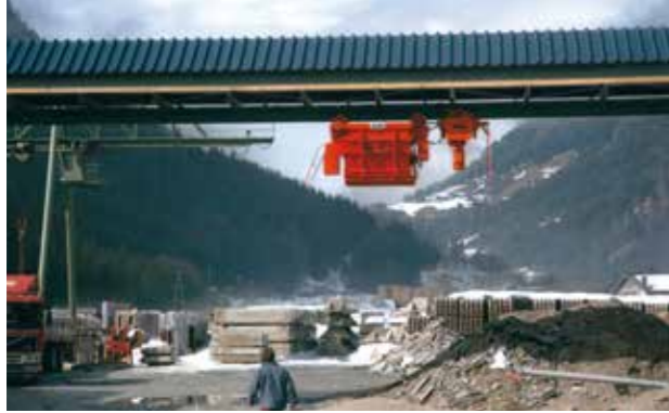
Flap bucket in a bridge 30 m
